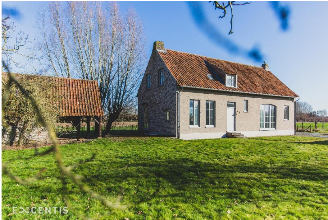
Figure 12 Outside view of the test house
